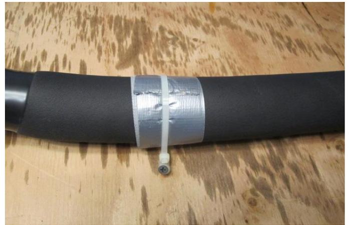
The duct line needs to be supported or it can crack the manifold and cause leaks. Wrap a couple of layers of duct tape before installing the zip tie strap to avoid damaging insulation.
